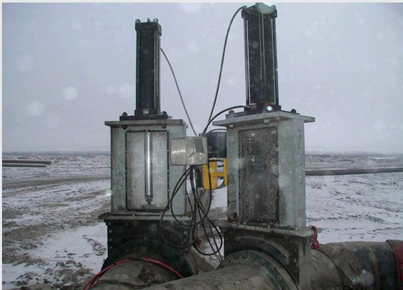
8" Bore ML Series with low temp seals
